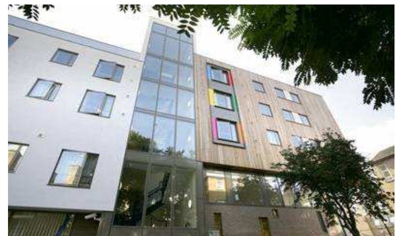
Somerset Court - Completed September 2006
